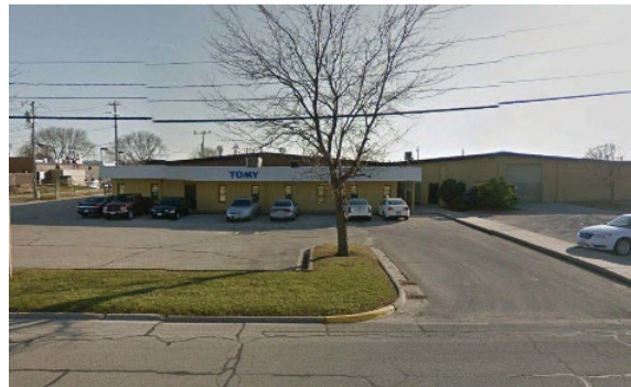
Looking south at the Property
